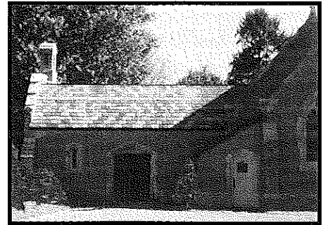
Exterior of new mausoleum
